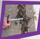
deterioration by hardening the asphalt, making susceptible it to cracking, as well as weathering away of the asphalt binder making the surface susceptible to raveling,
