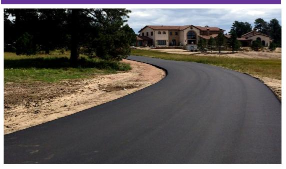
Asphalt pavement is a popular choice for residential driveways. Properly designed and constructed, it stays smooth, sound and attractive in appearance for many years. Flexibility allows the pavement to conform to minor settlements and still retain a continuous surface free of abrupt bumps. A well-designed, constructed and maintained driveway will give trouble-free service for up to 20 years and will add appeal and value to the property.
