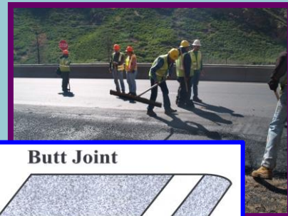
Papered Transverse Joint
