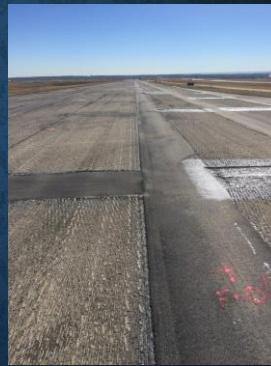
Cold Paving Joint
