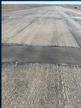
Wide Crack Repair
